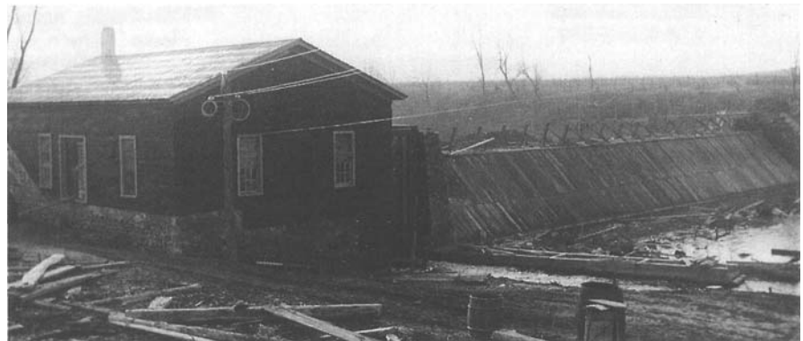
The 850-kW LaBarge Dam and Powerhouse, built in 1901 at the site of a sawmill, brought electricity and a more modern way of life to residents and local manufacturers of three communities in southwestern Michigan. (Photo courtesy Caledonia Historical Commission)
